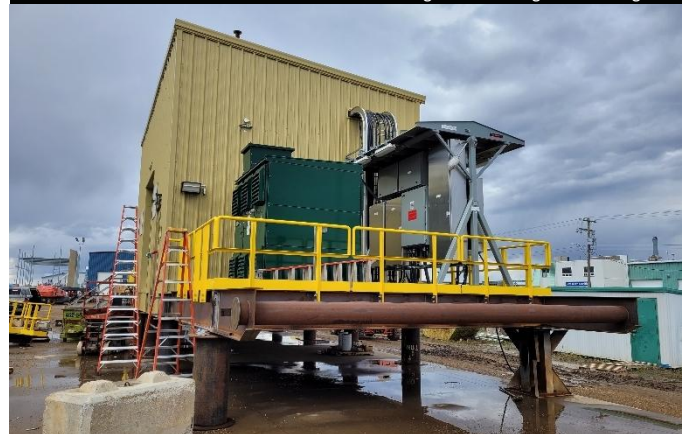
Air Bubbler Blower Building
