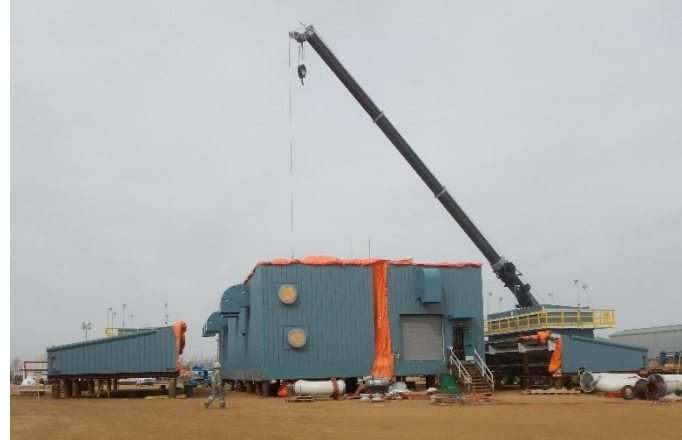
Modular Building Design – Tailing Pump Building
